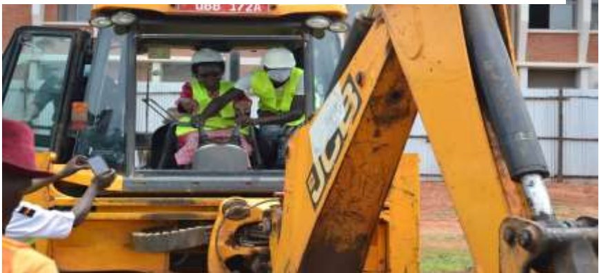
Figure 14 Hon. Dr. Jane Ruth Aceng Otero and other officials from MoH during the ground breaking for Lira satellite laboratory
