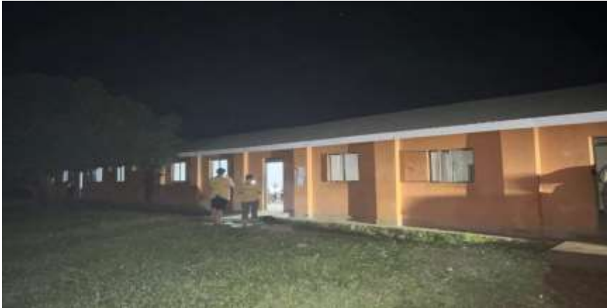
Figure 167 Nancy School for the Deaf after the installation of the solar light.
